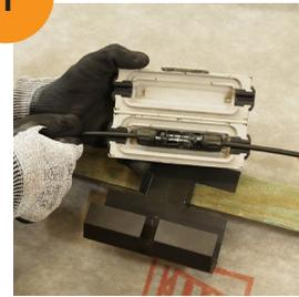
Place MC4 connector into enclosure with cables laid in grommet
