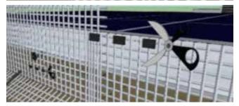
STEP 4: Cut off any excess mesh screen sticking over the top edge of the solar panel array. Cut of the clip assembly rod flush with the exterior of the speed washer. Use metal shears. Bird Barrier has them available.
