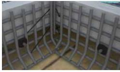
Inner Corner: Secure the first mesh panel in place so it butts up against the solar panel. Cut the bottom fold of the second mesh panel at a 45 degree angle so it does not interfere with the bottom bend of the first panel. Lock in place with Solar Panel Clips. Use zip ties if necessary to secure the two mesh panels together.
