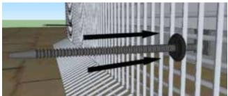
STEP 3: Slide the speed washer onto the shaft of the clip assembly until snug. Make adjustments to the screen as necessary. Tighten speed washer to panel edge.
