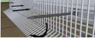
STEP 2: Set the wire mesh screen in place. Make sure the fastener rod comes through the screen at an upward angle as to keep downward pressure on the screen, pushing it towards the roof.
