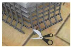
Outer Corner: Cut upwards from the bottom until the bend point. Bend the piece around the corner. Use zip ties, hog rings, or the Solar Clips to hold in place.
